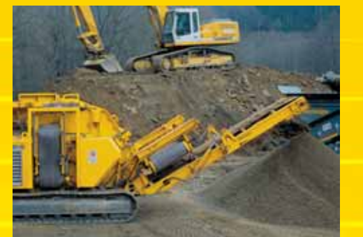
Making crushed material for pipe bedding
