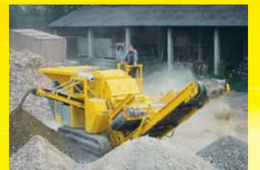
Recycling concrete with fine pre-screening
